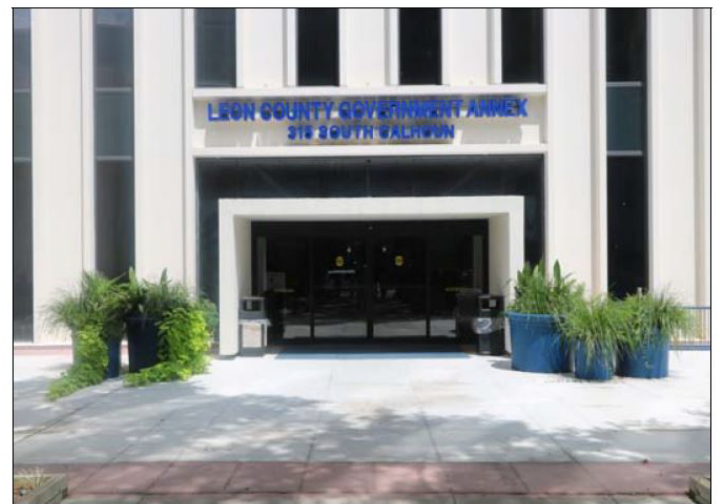
Leon County Government Annex Building
