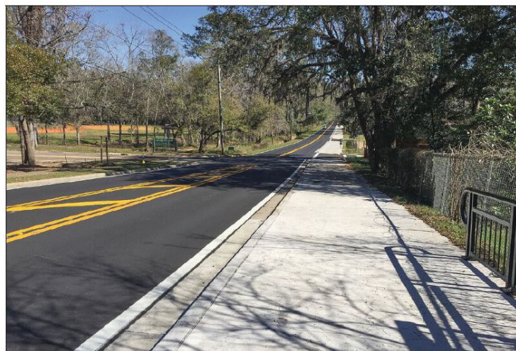
Local Road Resurfacing
