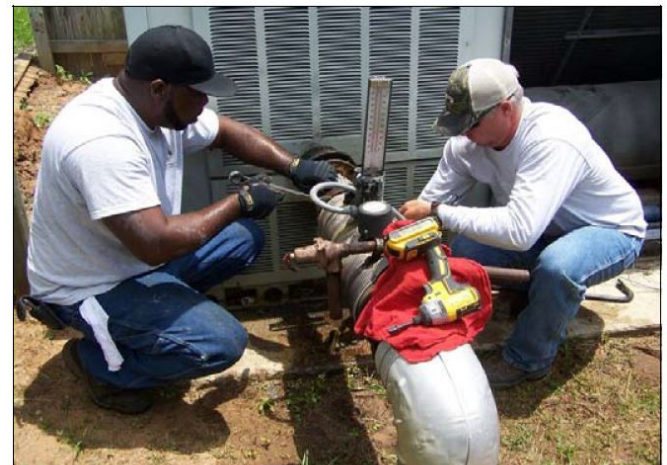
Building Mechanical Repairs and Improvements
