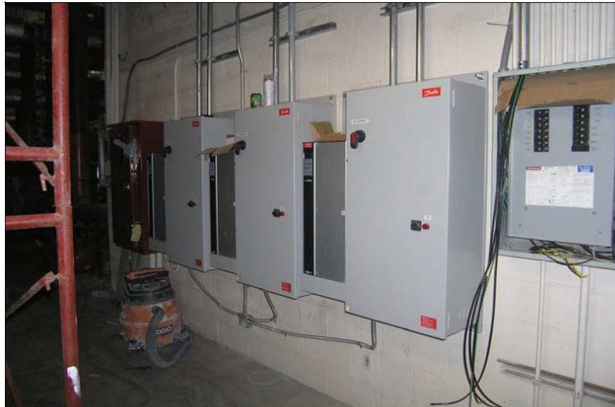
Architectural & Engineering Services- Electrical Panels
