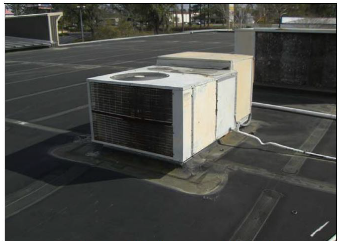
Building Roofing Repairs and Replacement
